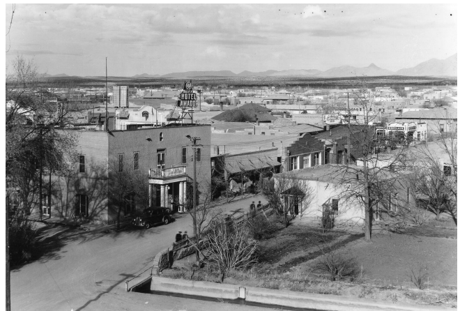
The Amador Hotel, ca. 1930s, currently under renovation, remains a legacy of Martin Amador and family. Image courtesy of NMSU Library and Special Collections.
