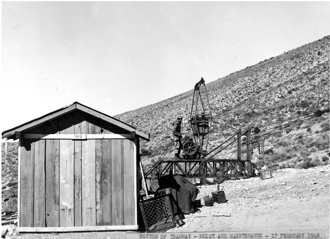
The tram base with a soldier in position to operate the tram. The small building was for storage and maintenance equipment. Shot on Feb. 17, 1948. Image courtesy of White Sands Missile Range.
